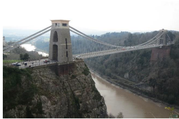
Clifton Suspension Bridge, Bristol
